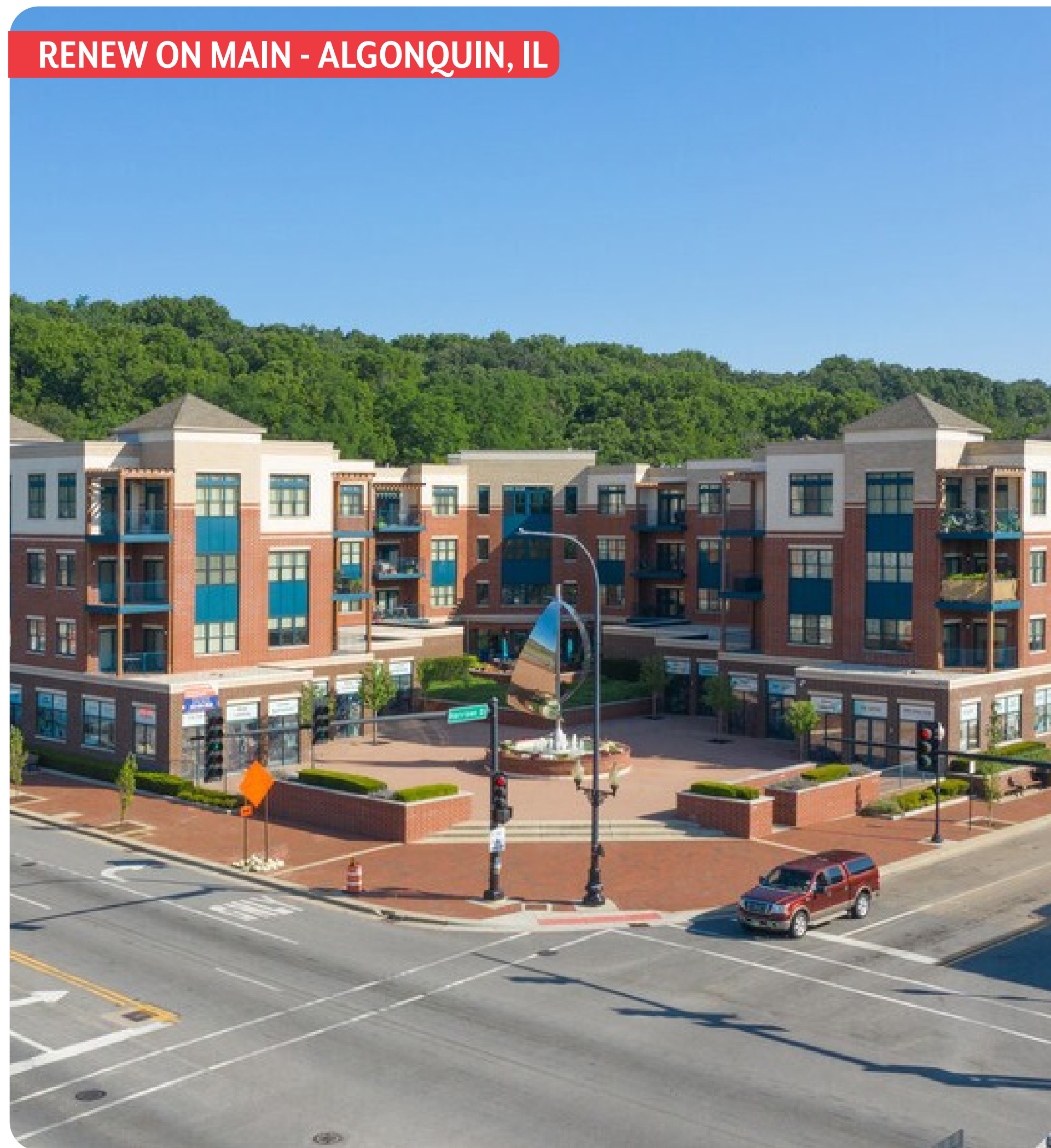
Downtown mixed-use development in Algonquin provides new retail and multi-family housing right downtown.
